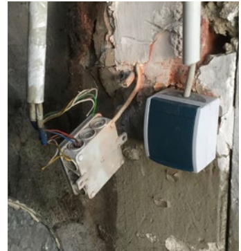
Abb. 6 Defekte Installation
